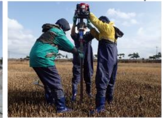
Gas-Power Core (gas pressure)
